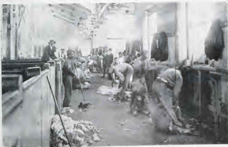
Shearing Sheep by Machinery, compressed air system at Wallington Lodge Station. S. J. Dailey photo.
