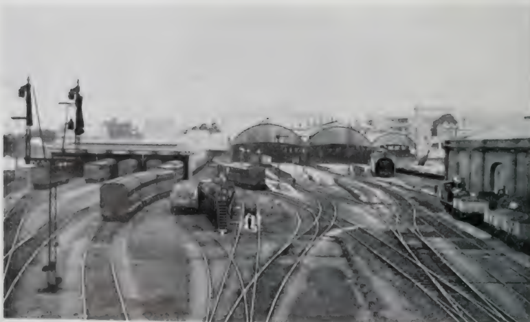
View from the Adelaide Railway Station. A. Vaughan, Survey Dept., photo.
