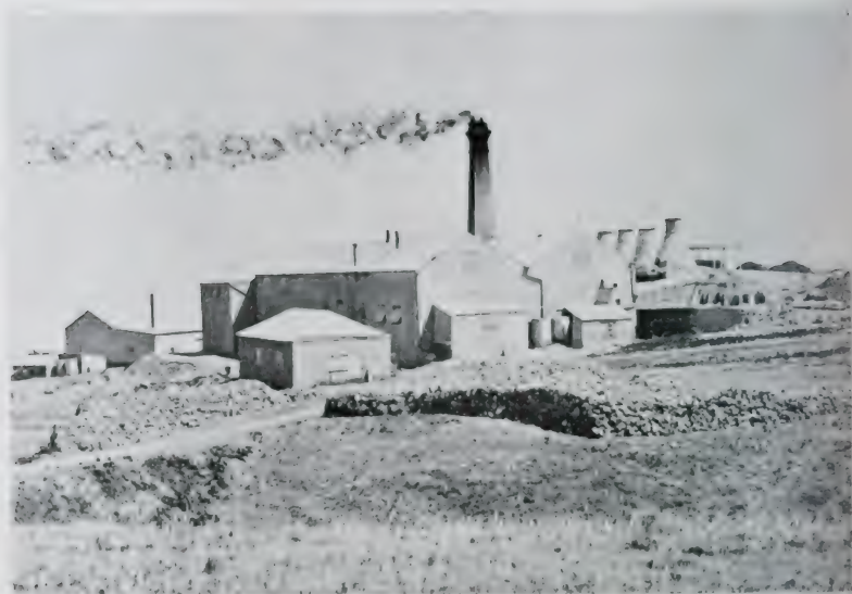
The Works of the S.A. Portland Cement Co., Ltd., Brighton.
