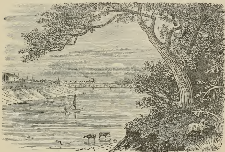
ILLINOIS CENTRAL RAILROAD BRIDGE AT DIXON, ILL.
