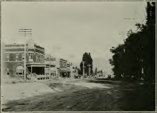
STATE STREET (Looking East).
