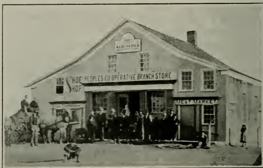
BUILDING OF LEHI UNION EXCHANGE.
