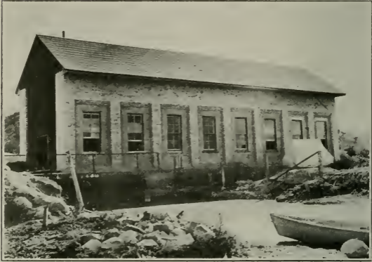
PLANT OF UTAH LAKE IRRIGATION COMPANY.
