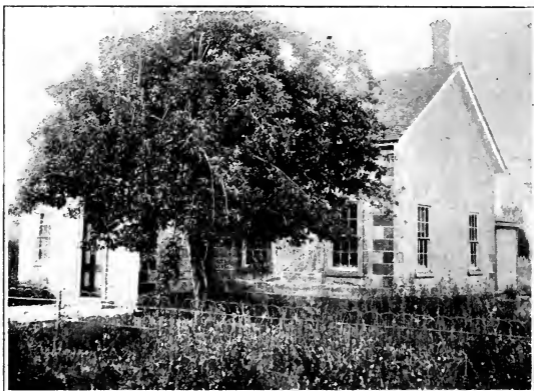
NEW WEST SCHOOL HOUSE.
