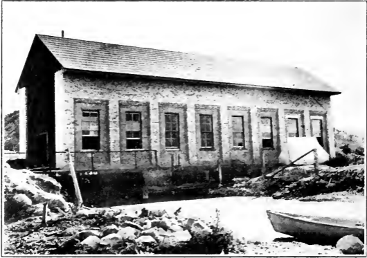
PLANT OF UTAH LAKE IRRIGATION COMPANY.
