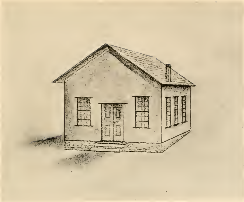
FIRST PRESBYTERIAN CHURCH, CEDAR RAPIDS, COMPLETED IN 1851
