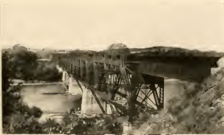
MILWAUKEE BRIDGE, AT COYINGTON
