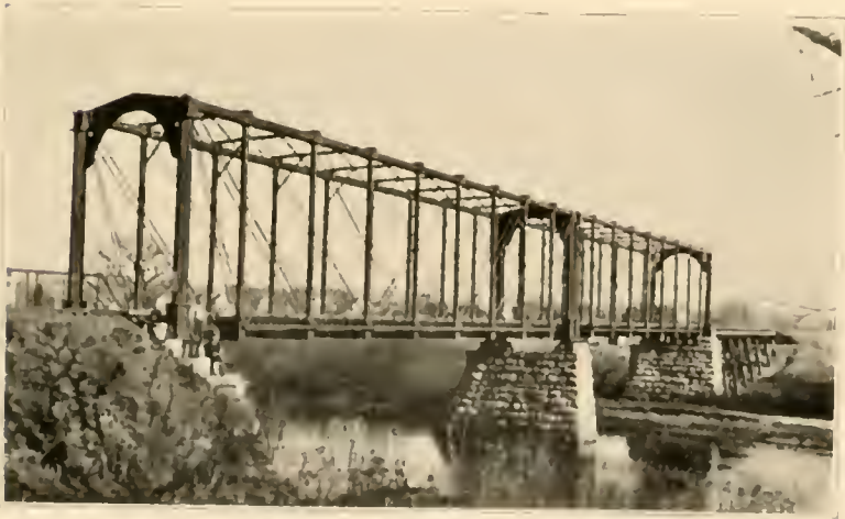
BRIDGE OVER WAISIE AT CENTRAL CITY
