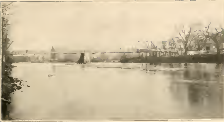
UPPER WAGON BRIDGE, CENTRAL CITY
