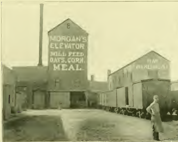
VIEW OF THOMAS MORGAN'S ELEVATOR AND YARDS.
