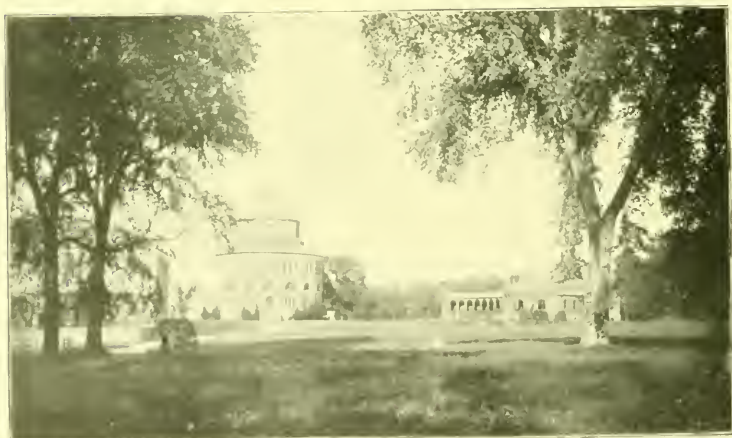
UNION COLLEGE, SCHENECTADY, N. Y. MEMORIAL HALL AND WASHBURN BUILDING.
