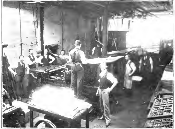
NEW HALL PRESS ROOM.
