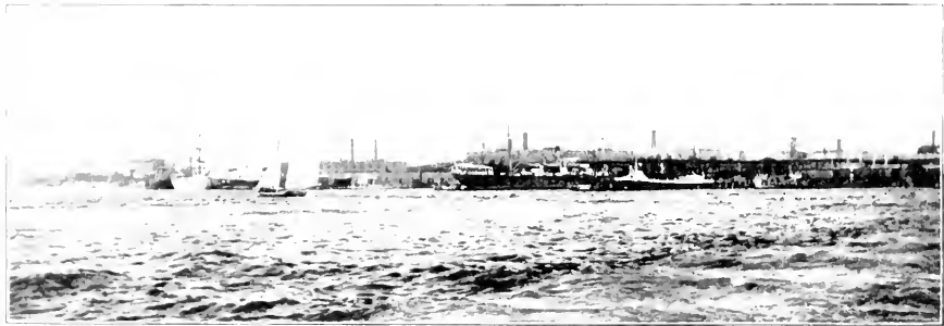
VIEW ON EAST FRONT, LONG ISLAND CITY.
