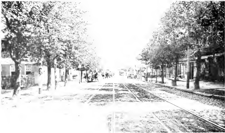
VIEW ON STEINWAY, E. 11TH AV., LONG ISLAND CITY.
