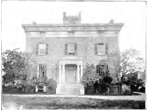
THE LONG ISLAND CITY HIGH SCHOOL (FORMERLY THE OLD 200' x 80' MANSION.)
