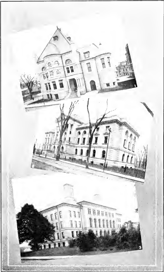
1 MEMORIAL BUILDING AND PUBLIC LIBRARY 2 MIDDLESEX COUNTY COURT HOUSE 3 STATE NORMAL SCHOOL
