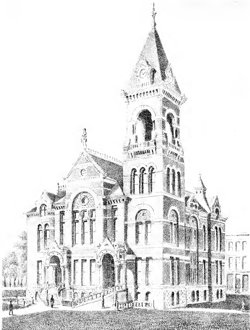
MACOMB COUNTY COURT HOUSE, 1881-2.
