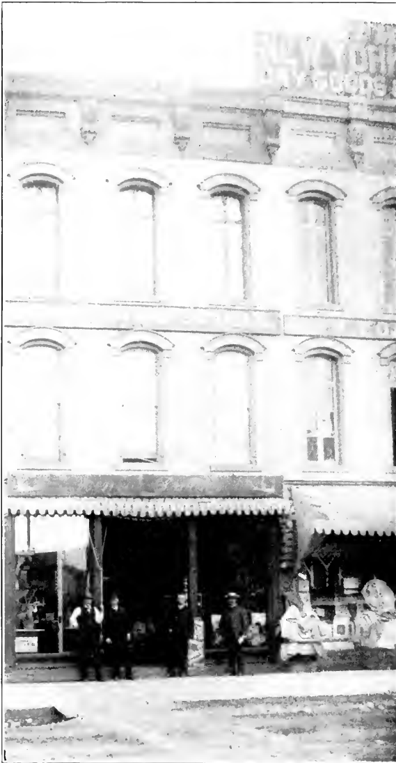
CARTER AND STAPP BUILDINGS 139 North Water Street
