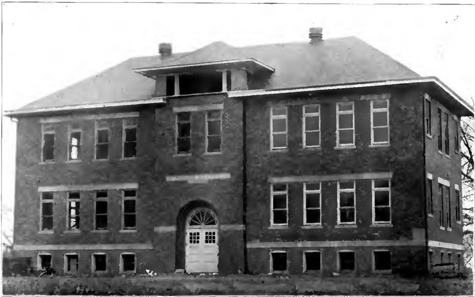
NEW HIGH SCHOOL BUILDING, PALMYRA
