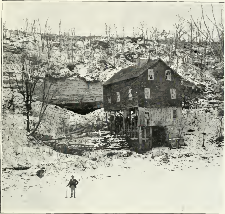
BACKBONE MILL, LINCOLN TOWNSHIP
