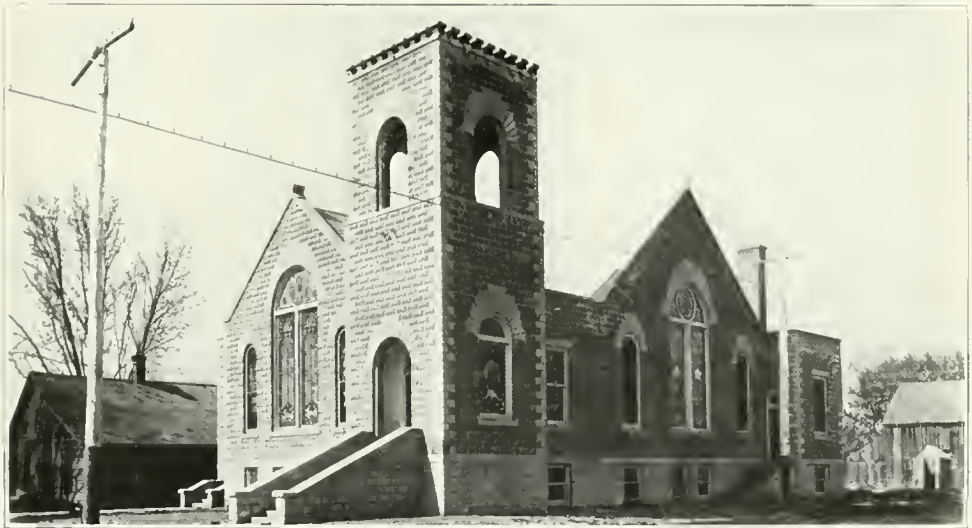
NEW METHODIST EPISCOPAL CHURCH, EARLIHAM
