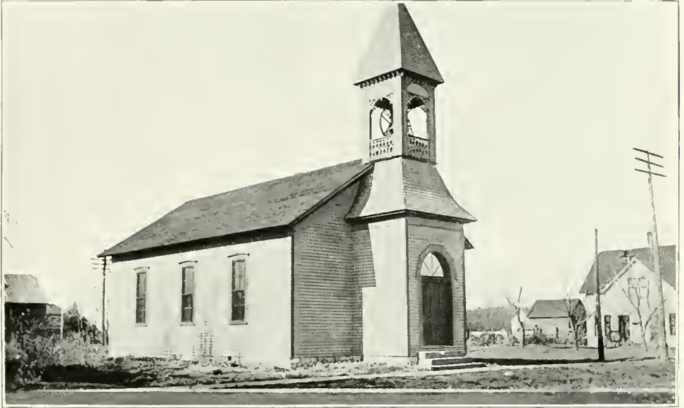
OLD METHODIST EPISCOPAL CHURCH, EARLIHAM
