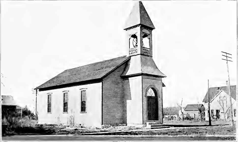
OLD METHODIST EPISCOPAL CHURCH, EARLIHAM
