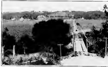
AFTON ROAD BRIDGE, LOOKING NORTH, LINCOLN TOWNSHIP
