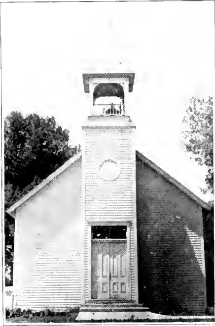
METHODIST CHURCH, MACKSBURG Built and dedicated in 1876. Repaired, re- modeled and rededicated in 1914
