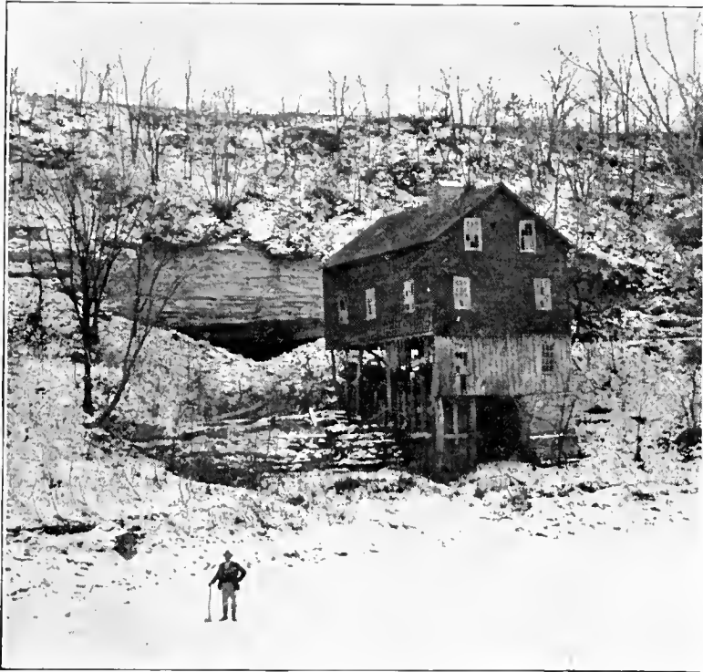
BACKBONE MILL, LINCOLN TOWNSHIP
