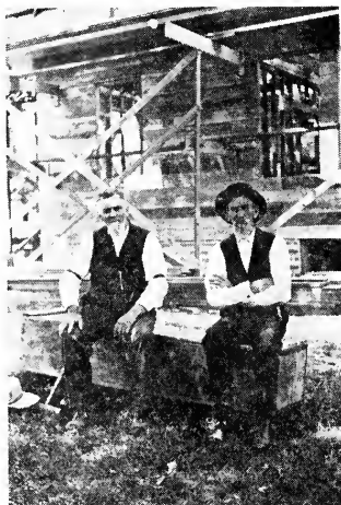
Building of Bryan House Robert Davis and R. G. Rayburn
