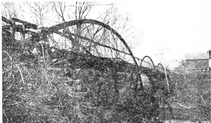
Bridge Over Sangamon River East of Mahomet At top, Sam Stout, below, Roscoe Lindsey
