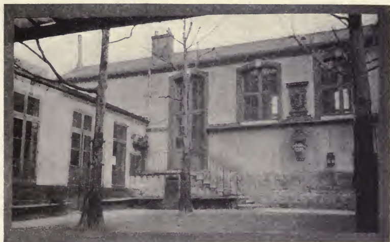
FIG. 45. WORKSHOP BUILDING, SALICIS SCHOOL
