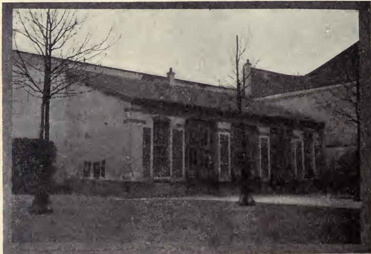
FIG. 58. WORKSHOP BUILDING, PUBLIC SCHOOL, RUE ST. MAUR
