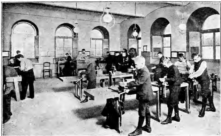
FIG. 36. METAL SLOYD ROOM, STOCKHOLM
