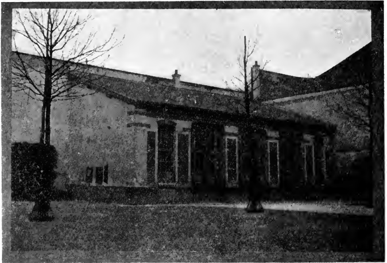
FIG. 58. WORKSHOP BUILDING, PUBLIC SCHOOL, RUE ST. MAUR
