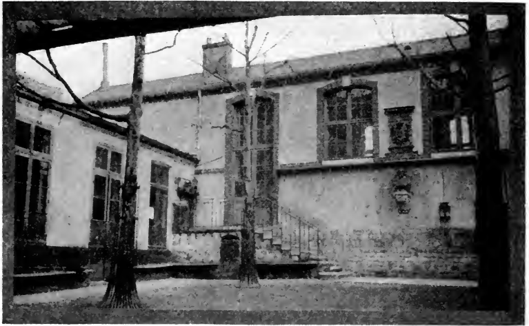
FIG. 45. WORKSHOP BUILDING, SALICIS SCHOOL
