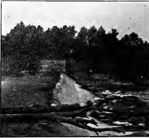
The (former) Wabash Canal Feeder Dam Across the River St. Joseph six miles above Fort Wayne. This is the Highest Dam in the Maumee River Basin, the water here shown in lower stage falling fifteen feet upon the Apron. Looking north of east 14th July, 1902. The former Feeder Canal, beginning just above this view, is now used by the Fort Wayne Electric Light and Power Company for water power.
