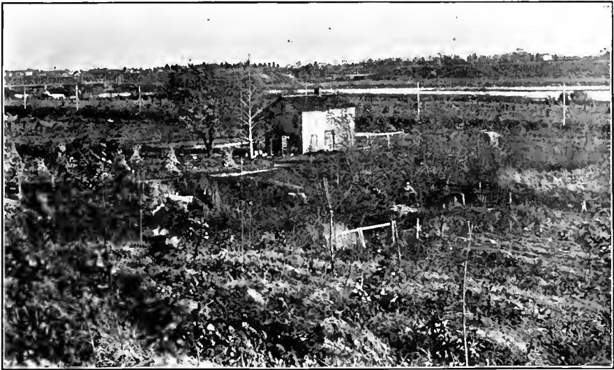
SITE OF FORT MEIGS FROM OPPOSITE SIDE OF RIVER.
