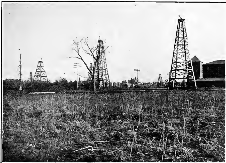
Edge of the Petroleum District, Findlay, Ohio, one mile north of the Blanchard River. Looking southeast 1st May, 1902. The Lake Erie & Western Railway in foreground. Manufactory of Fire-clay Pots on right. Petroleum wells being pumped under the Derricks which serve as supports for the Drills. Ward School Building to right of center, and tower of Findlay College between cluster of Derricks and telegraph pole to left of center.
