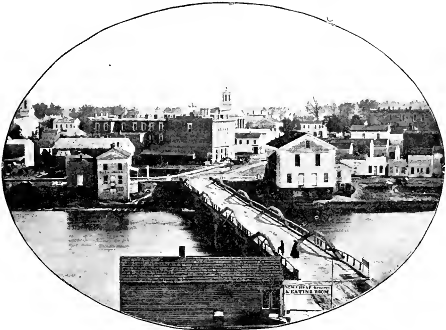
THE VILLAGE OF DEFIANCE IN 1868 LOOKING SOUTH
