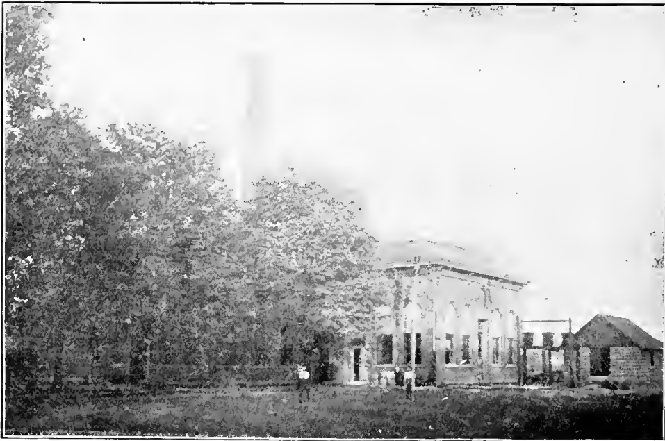
WATER WORKS PUMPING STATION
