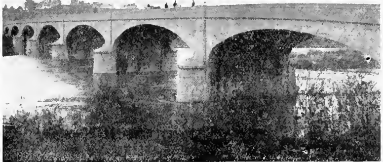
CONCRETE BRIDGE OVER WABASH RIVER, PERU
