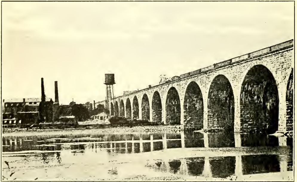
PENNSYLVANIA RAILROAD BRIDGE, NEW BRUNSWICK
