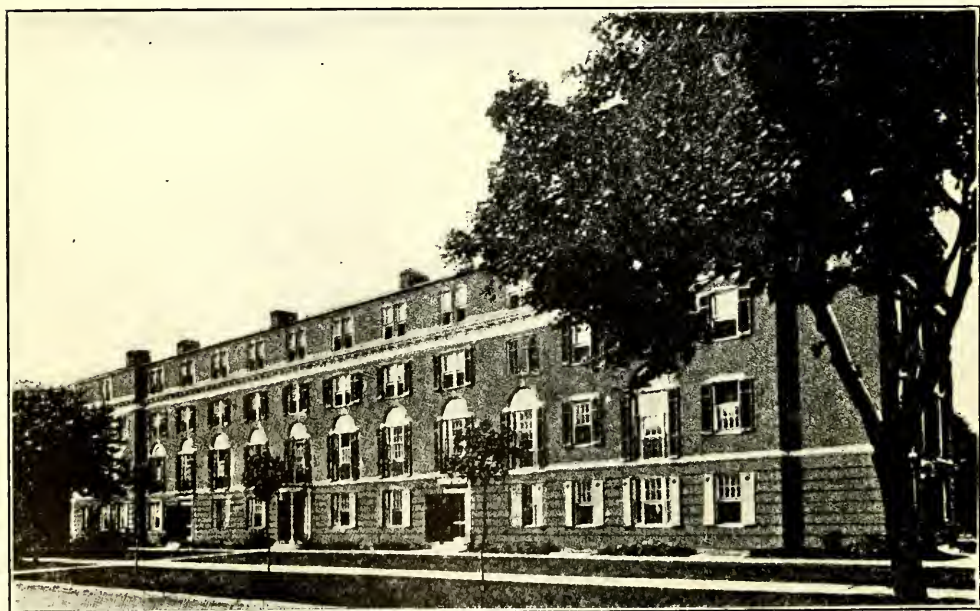
RUTGERS COLLEGE FORD DORMITORY—ENGINEERING BUILDING
