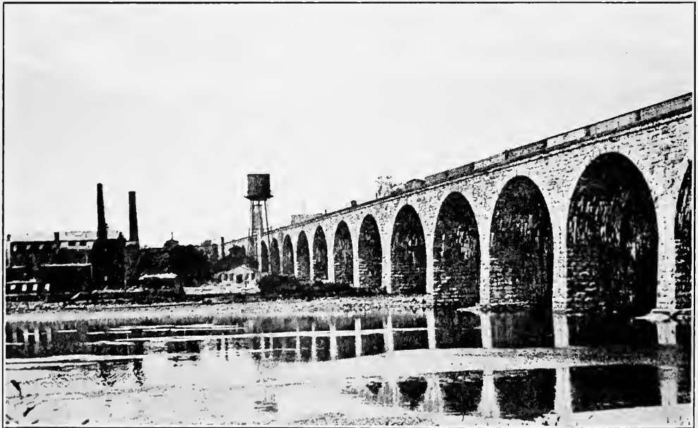
PENNSYLVANIA RAILROAD BRIDGE, NEW BRUNSWICK
