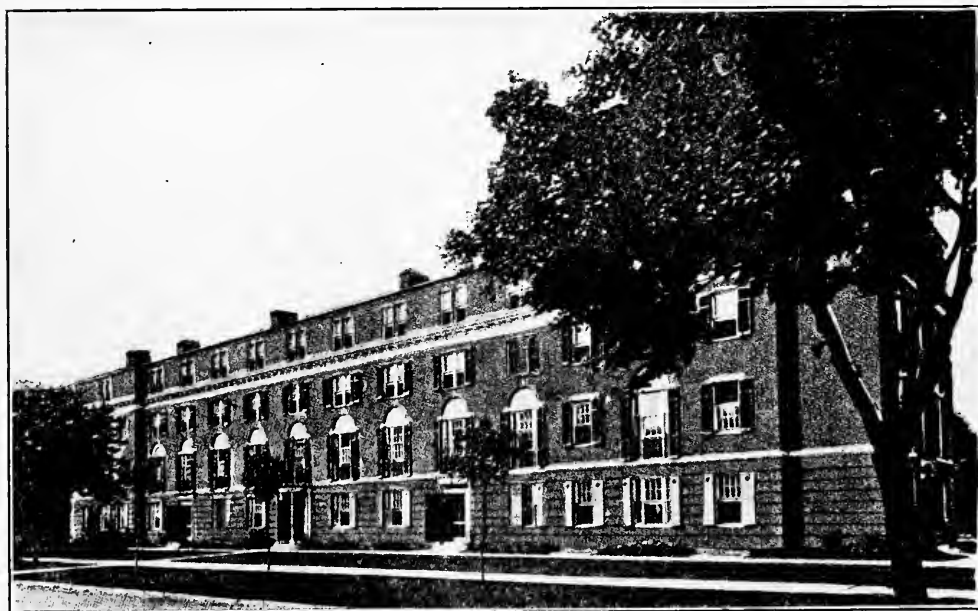
RUTGERS COLLEGE FORD DORMITORY—ENGINEERING BUILDING
