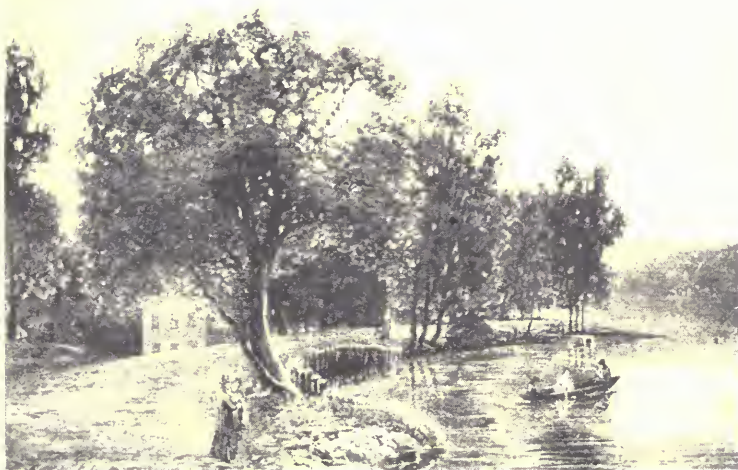
CHOUTEAU'S POND AND DAM
