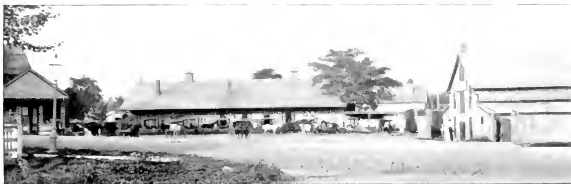
THE STATION, NEW YORK RAILROAD.
