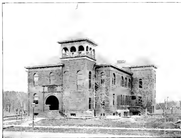
NEW SCHOOL BUILDING.
