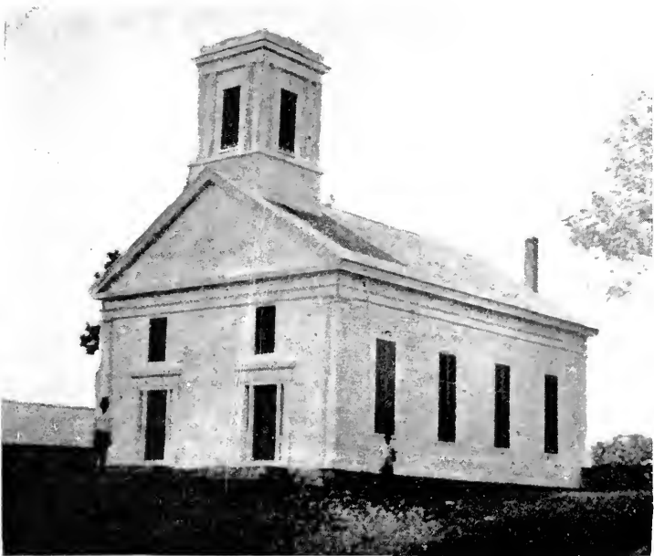
CONGREGATIONAL CHURCH (MONTVILLE CENTER).
