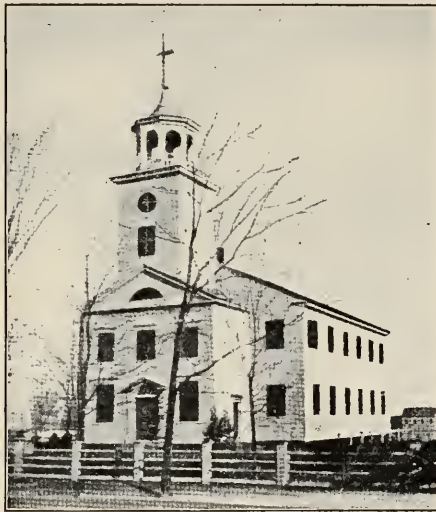
FOURTH PARISH MEETING HOUSE IN NEWBURY, 1816.
