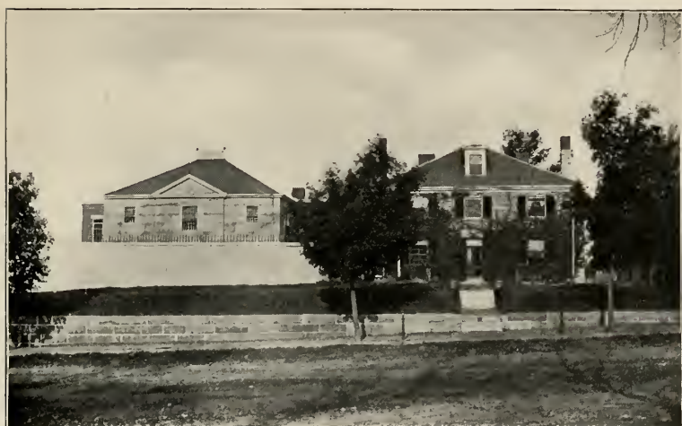
JAIL AND JAIL-KEEPER'S HOUSE.
