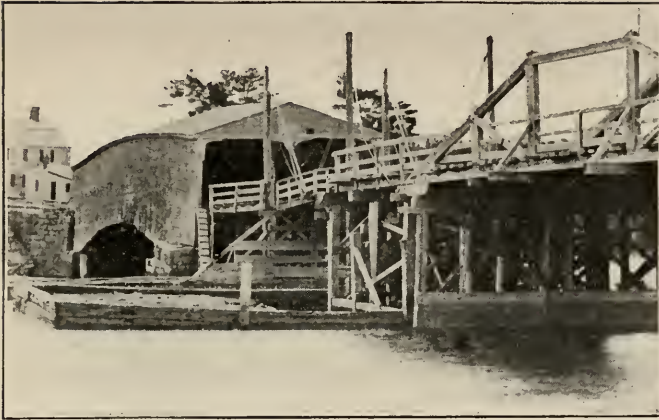
BRIDGE FROM DEER ISLAND TO SALISBURY, 1792.
