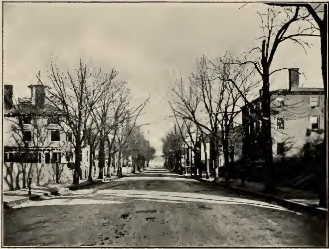
VIEW OF GREEN STREET FROM HIGH STREET.
