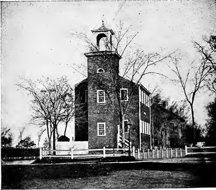
SCHOOLHOUSE AT SOUTHEASTERLY END OF BARTLET MALL.
