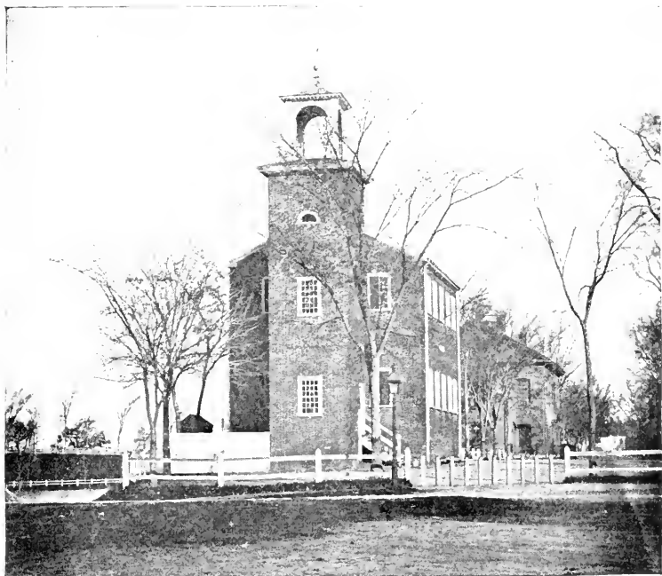
SCHOOLHOUSE AT SOUTHEASTERLY END OF BARTLET MALL.
