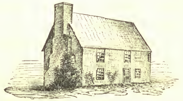
Whitefield’s House, as seen from the west.
