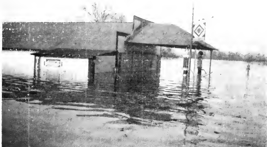
Henry Sparrow Garage During Flood January, 1937
