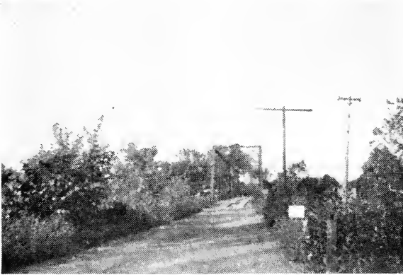
Picture of Bridge Across Little Wabash
