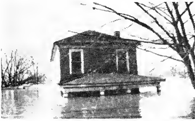
Andrew Bosaw Residence February 6, 1937. Water Had Dropped 1½ Ft.
