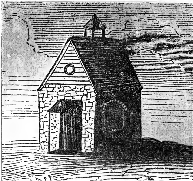
THE FIRST STONE CHURCH AT NEW PALTZ
