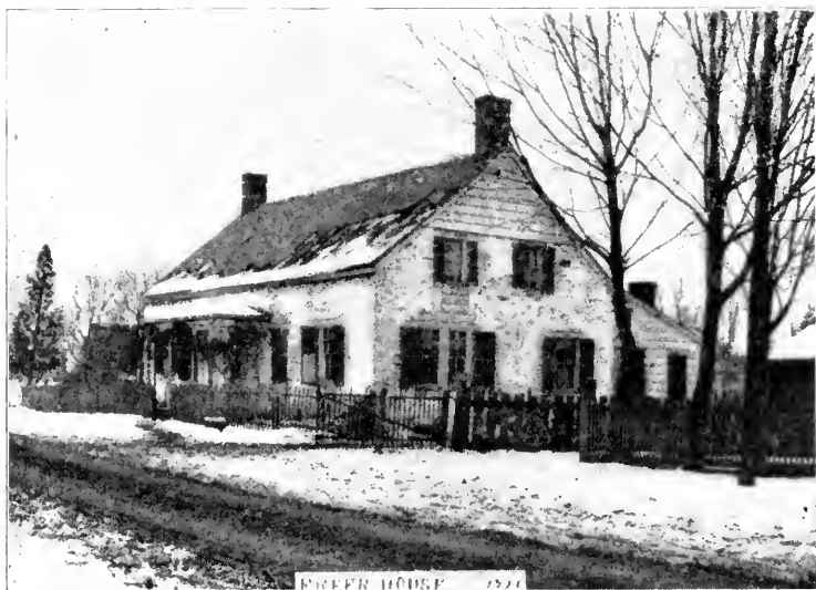
THE OLD FREER HOUSE AT NEW PALTZ
