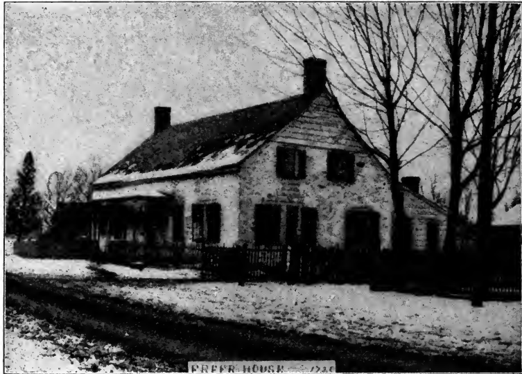
THE OLD FREER HOUSE AT NEW PALTZ
