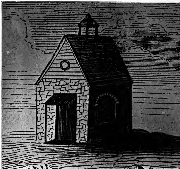
THE FIRST STONE CHURCH AT NEW PALTZ
