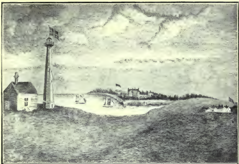
LIGHTHOUSE AND LIGHTHOUSE KEEPER'S HOME, BUILT 1803.
