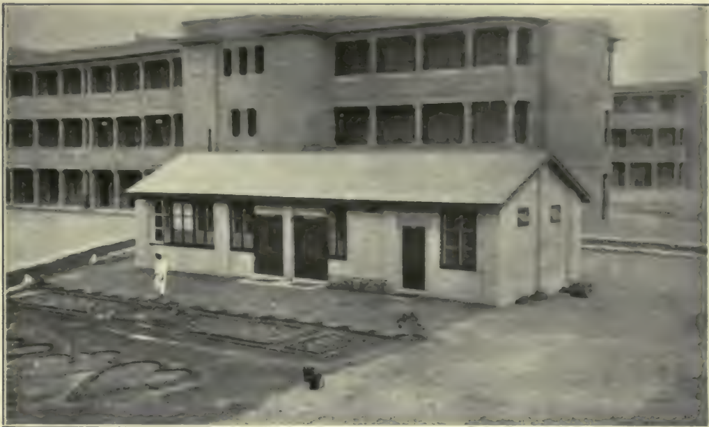
OPERATING THEATRE, X-RAY DEPARTMENT, LABORATORY, AND BLOCK I., CAIRO.
