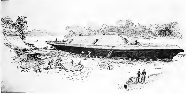
CONSTRUCTION OF THE ALBEMARLE
