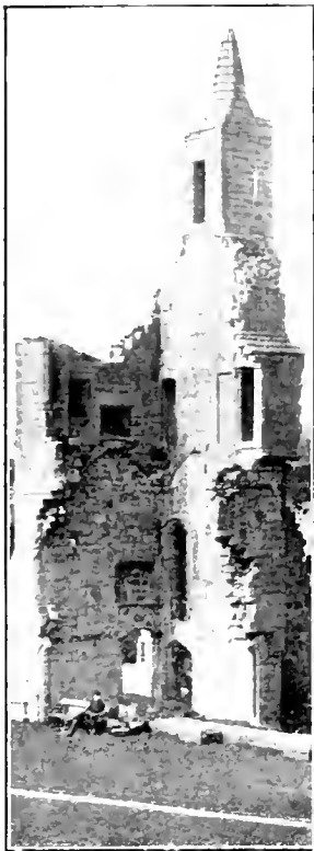
THE LITTLE STAIR TOWER.
