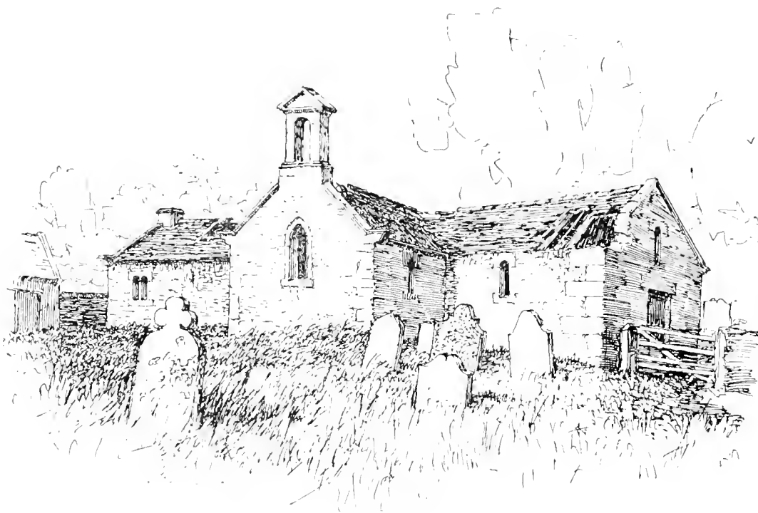
SHOTLEY CHURCH, JULY 3RD, 1882. 2
