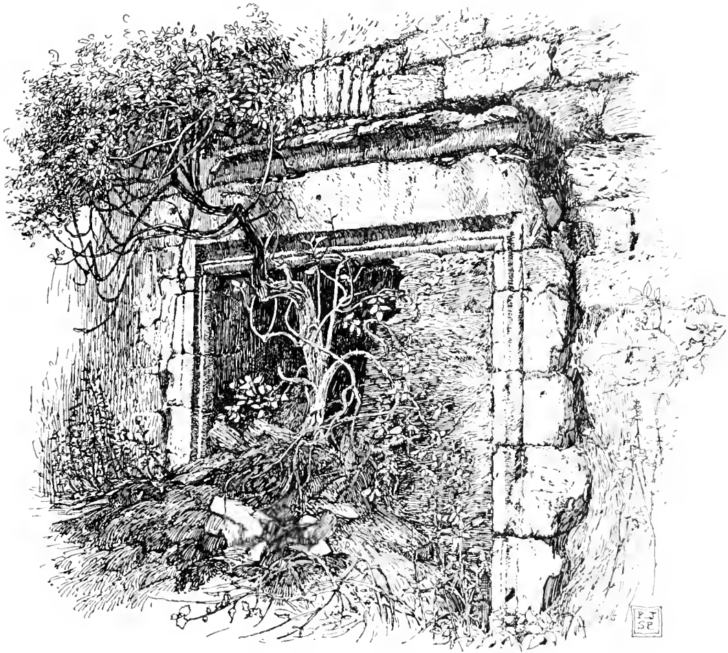
FIREPLACE IN LEMINGTON TOWER.
