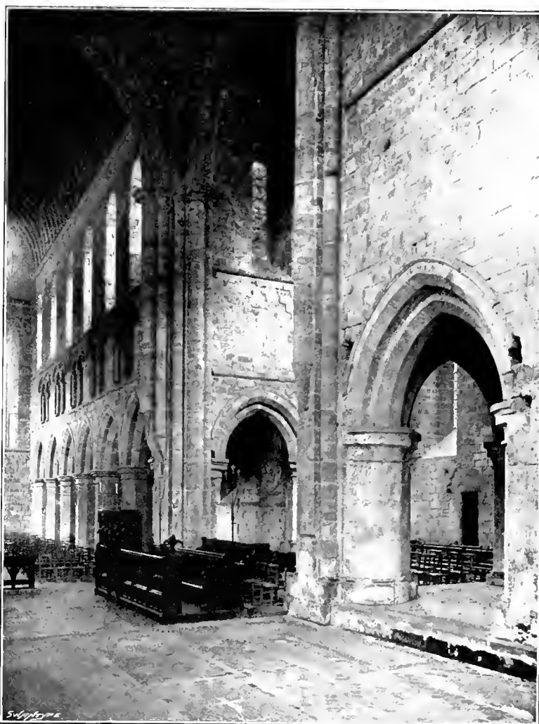
INTERIOR OF THE CHURCH (looking west).
