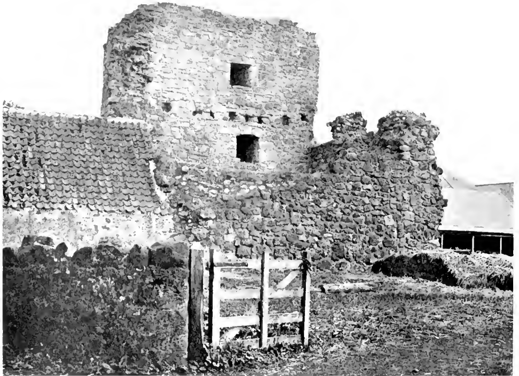
FIG. 8. HOWTEL TOWER FROM THE NORTH-EAST.
