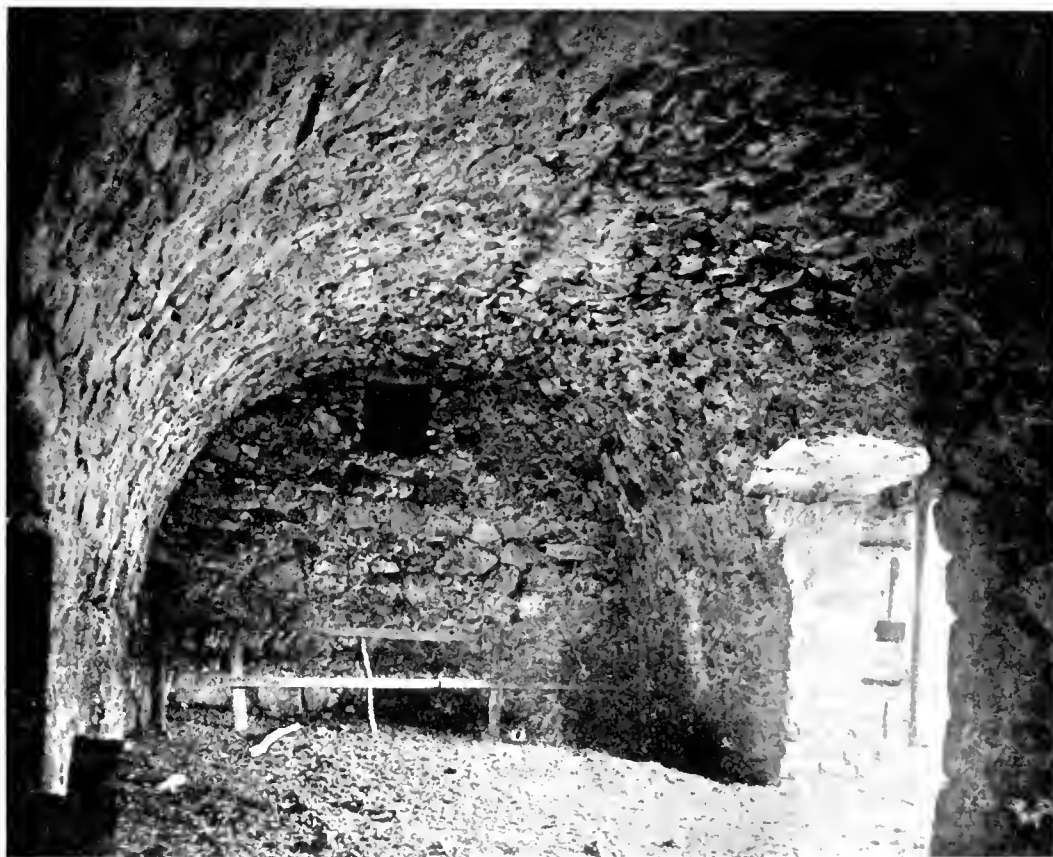
FIG. 11. INTERIOR OF BASEMENT, AKELD TOWER.
