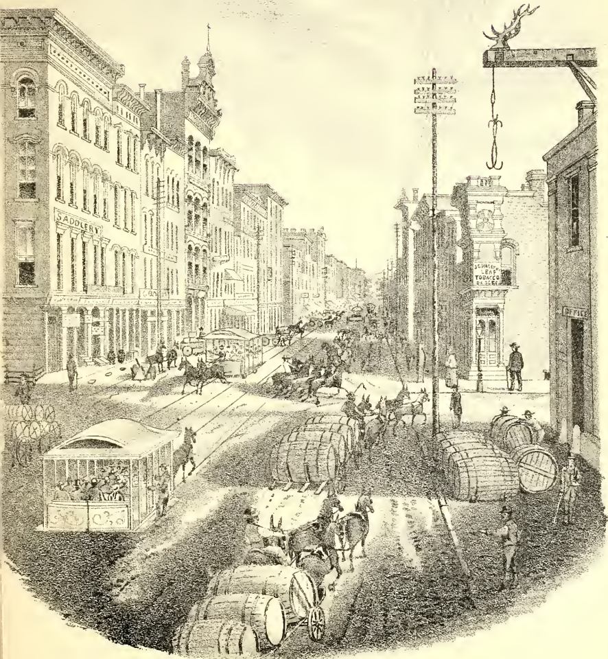
VIEW OF MAIN STREET, LOOKING EAST. LOUISVILLE, KENTUCKY.
