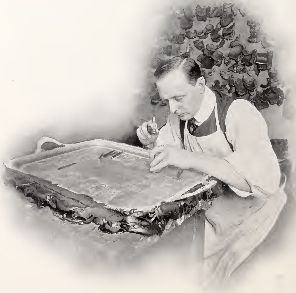
Illustration of the process of Chasing.
