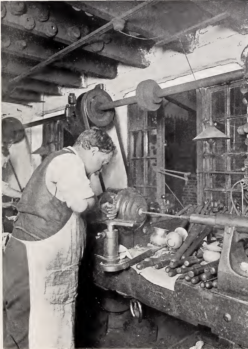
Illustration of Spinning.
