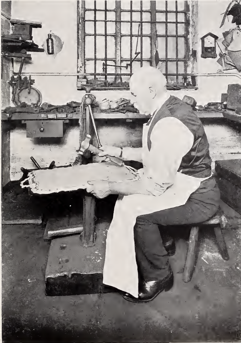
Illustration of Flat Hammering.
