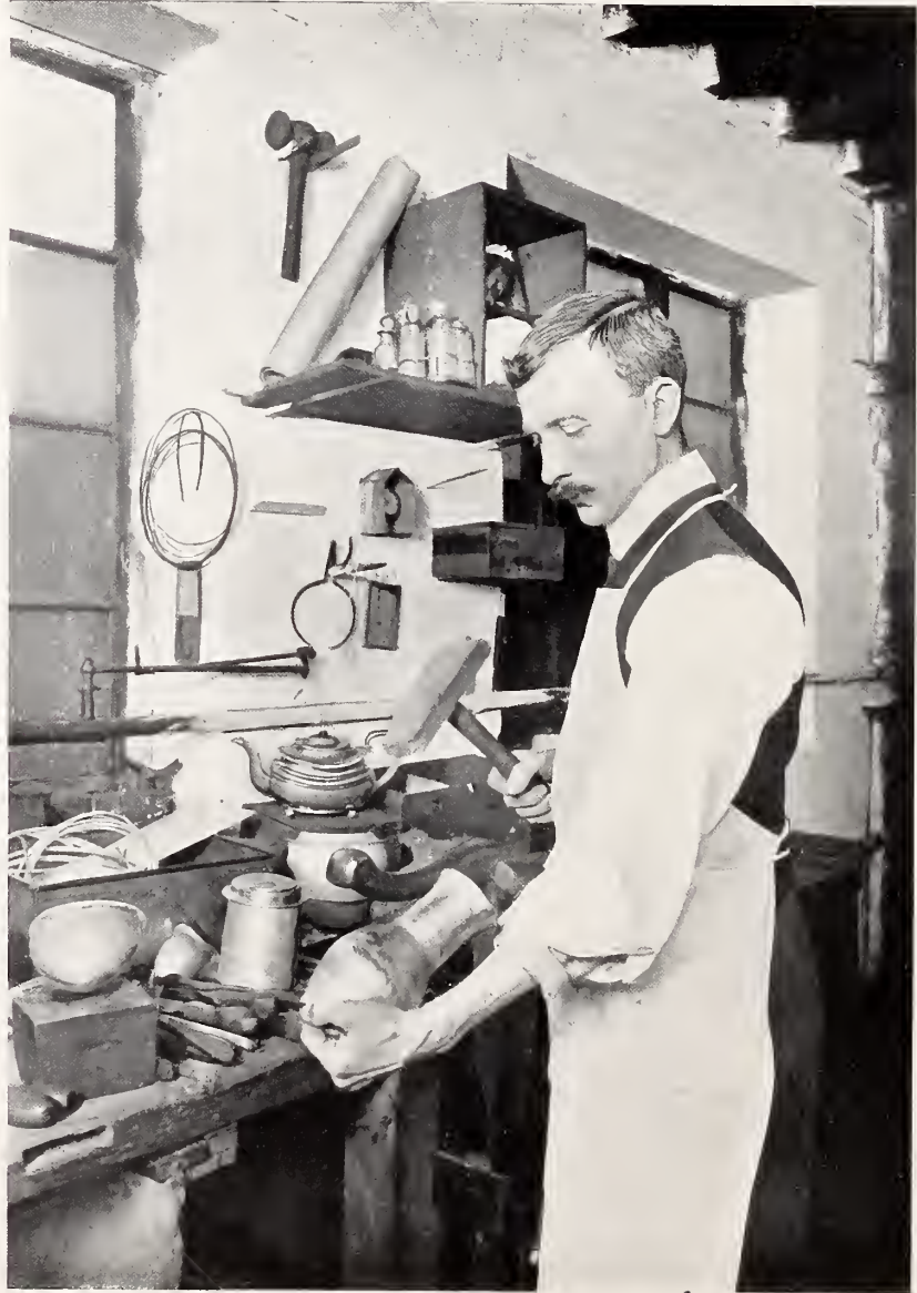
1.—Illustration of Raising by Hand.
