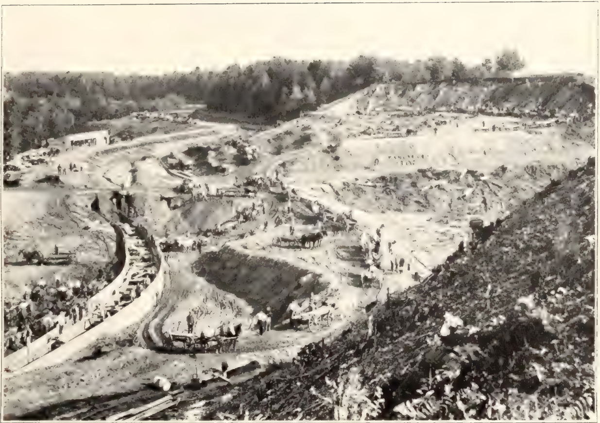
REPAIRING THE GREAT BREAK IN THE BLACK RIVER CANAL AT FORESTPORT
