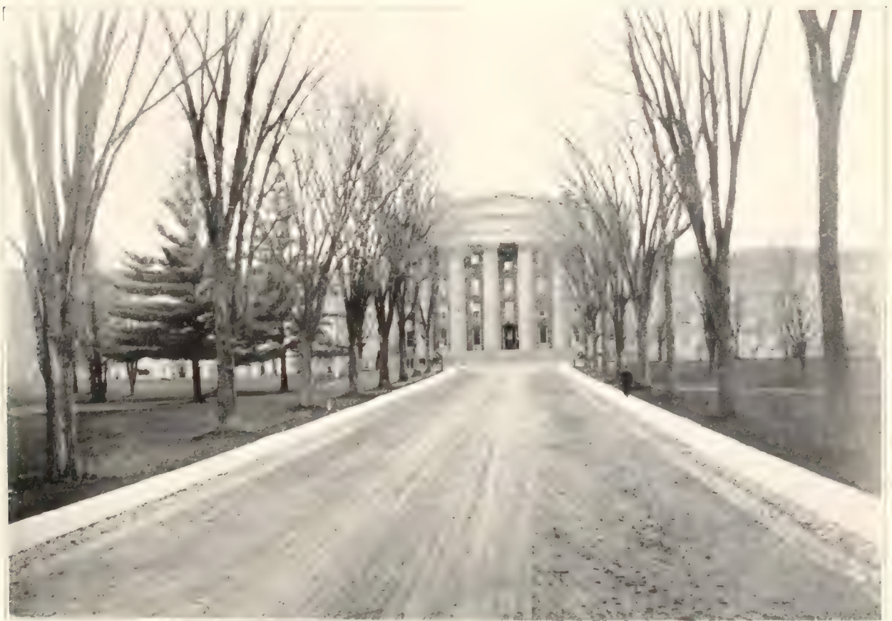
APPROACH TO THE NEW YORK STATE HOSPITAL AS IT NOW APPEARS
