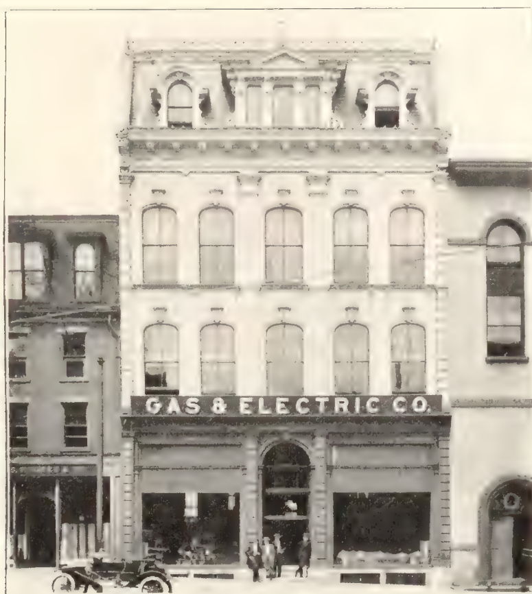
THE OLD COUNTY CLERK'S OFFICE IN UTICA, NOW THE UTICA GAS & ELECTRIC COMPANY'S OFFICES
