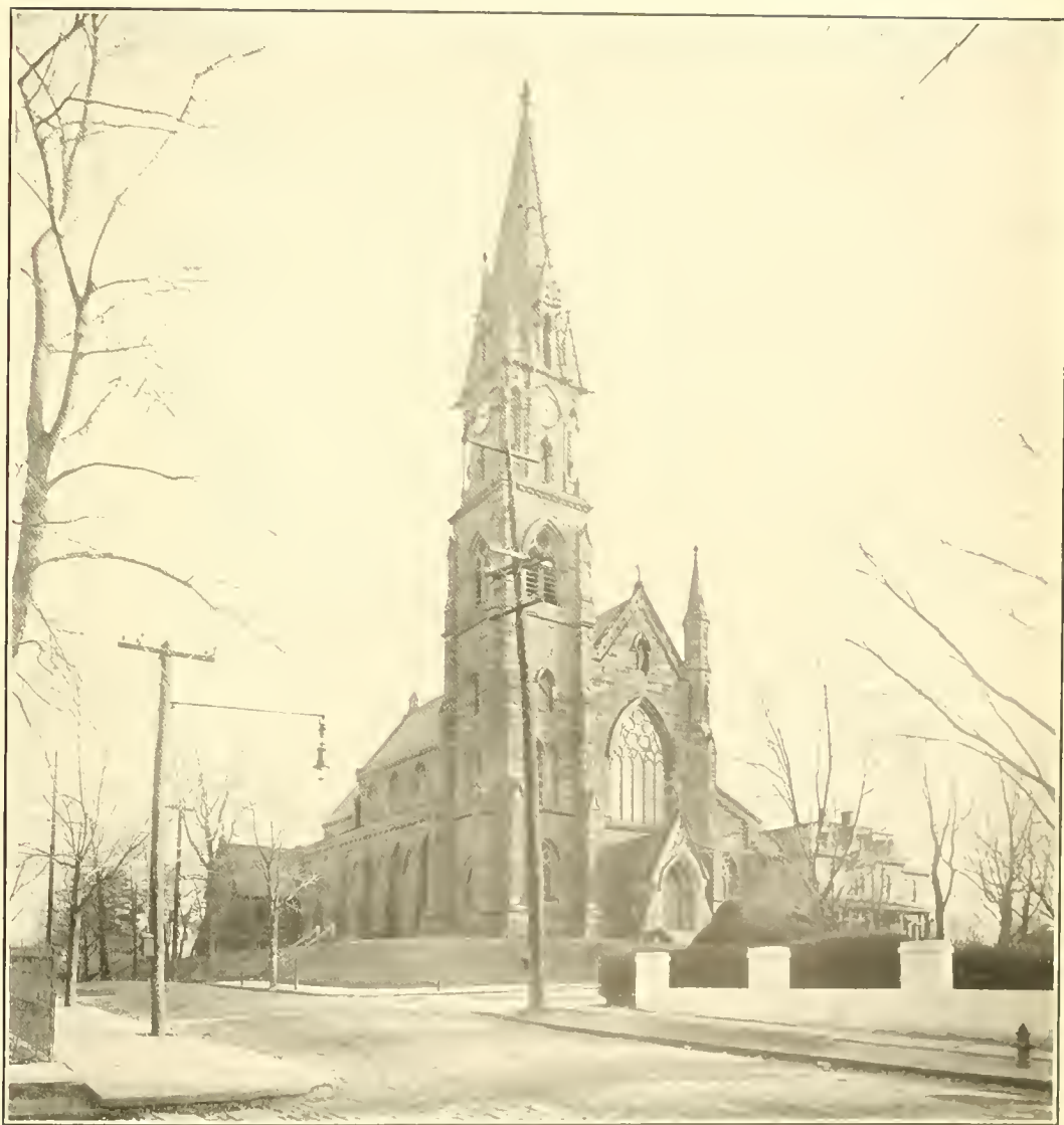
ST. JOHN'S CATHOLIC CHURCH, EDGE AND WILCOX STS., ORANGE
