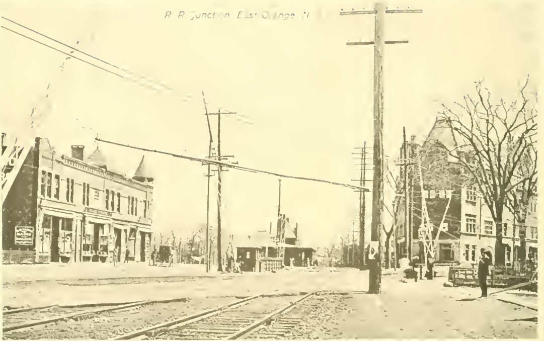
RAILROAD JUNCTION, EAST ORANGE
