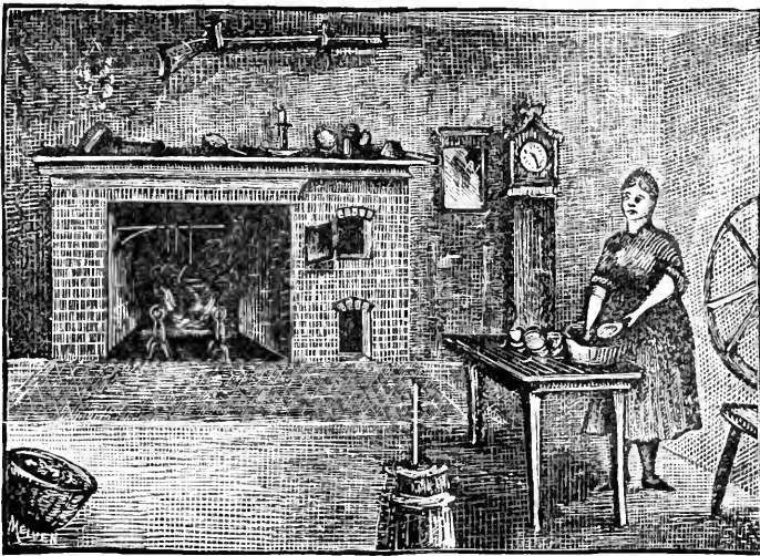
FIREPLACE IN BRICK CHIMNEY.
