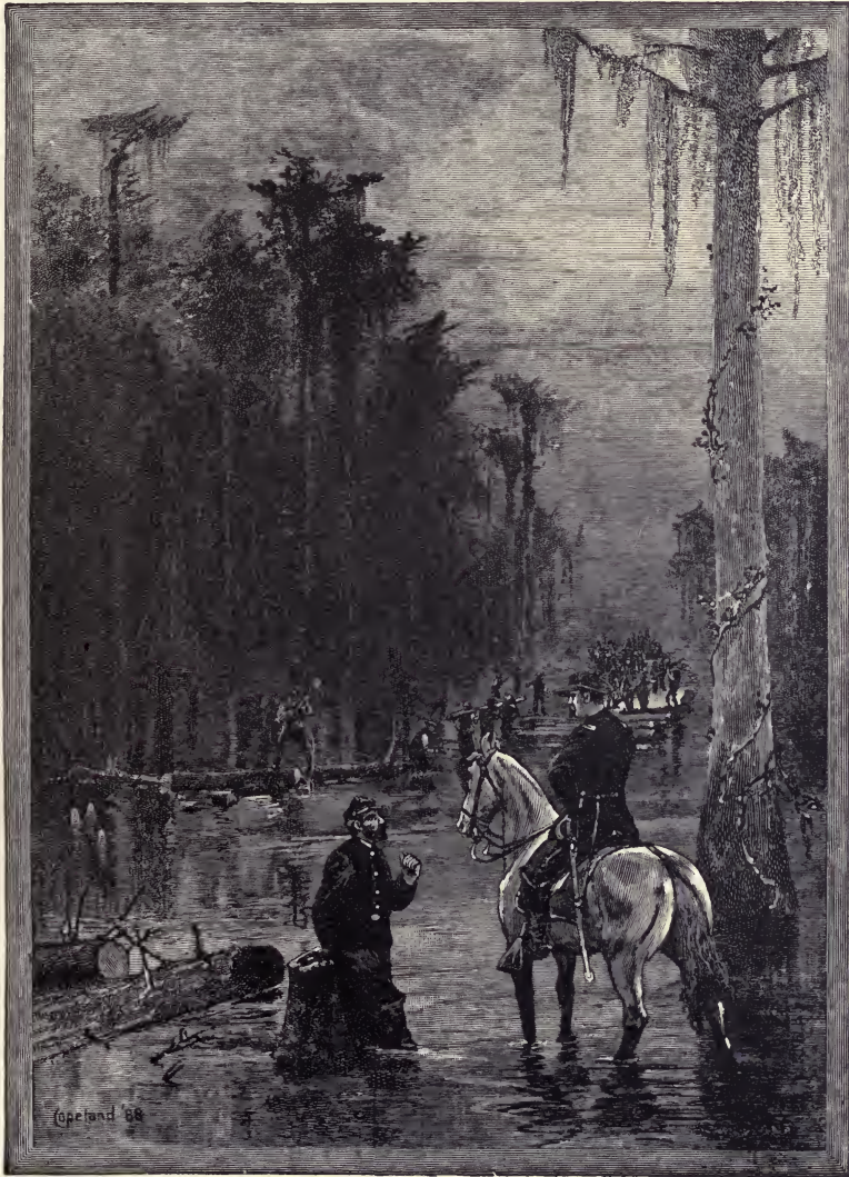
CONSTRUCTING A MILITARY ROAD THROUGH THE SWAMPS
