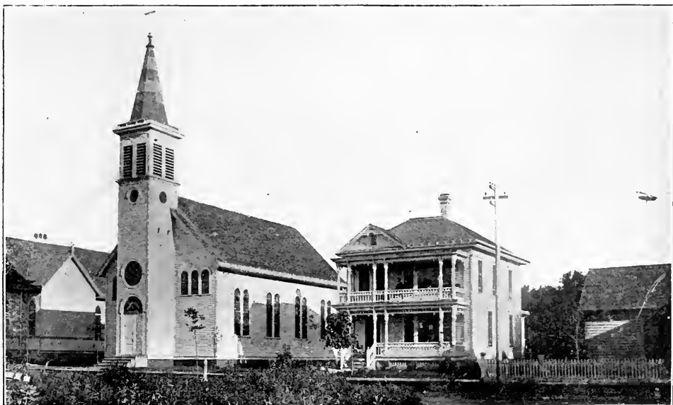
ST. MARY'S CATHOLIC CHURCH, SHENANDOAH
