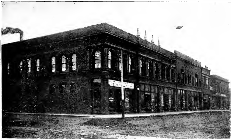
SHERIDAN AVENUE WEST FROM SYCAMORE, SHENANDOAH
