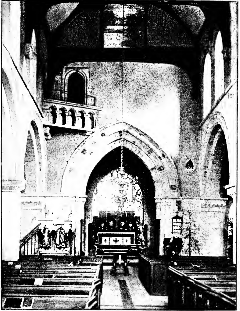
WESTERN TOWER ARCH.
