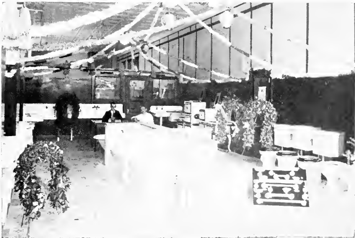
FRONT—OFFICES, SHOW ROOMS AND STOCK ROOMS
