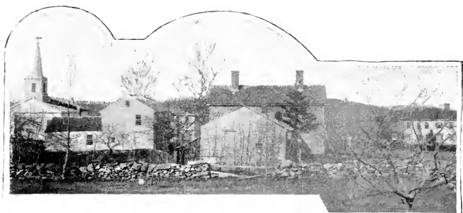
PELHAM CENTER FROM THE SOUTH.
