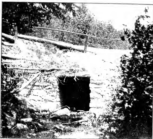
STONE BRIDGE OVER THE DUNLAP BROOK.
