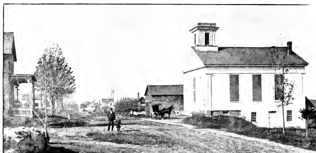
METHODIST CHURCH, WEST PELHAM.
