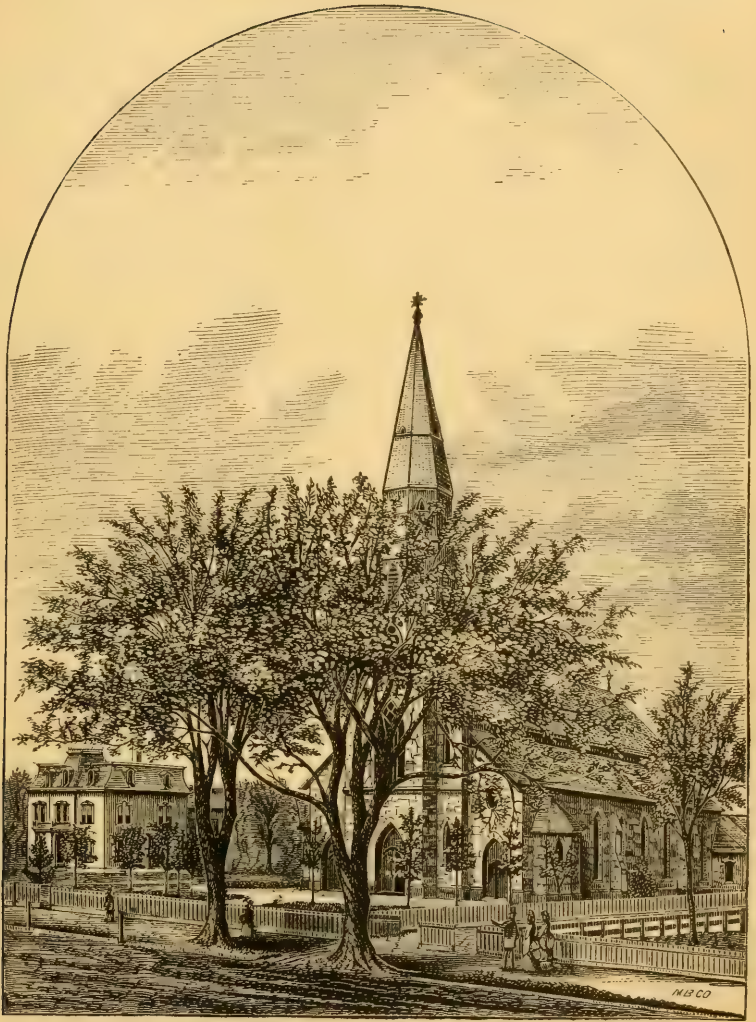
ST. JOSEPH'S R. C. CHURCH AND RESIDENCE OF PASTOR.
