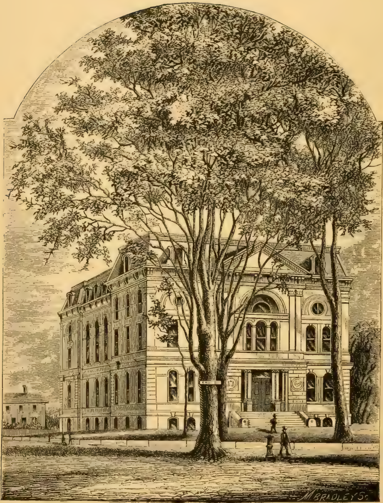
BERKSHIRE COUNTY COURT HOUSE.
