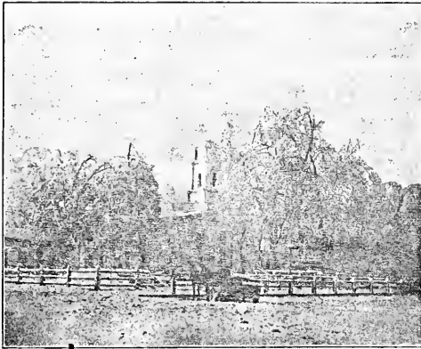
OLD COURT HOUSE
