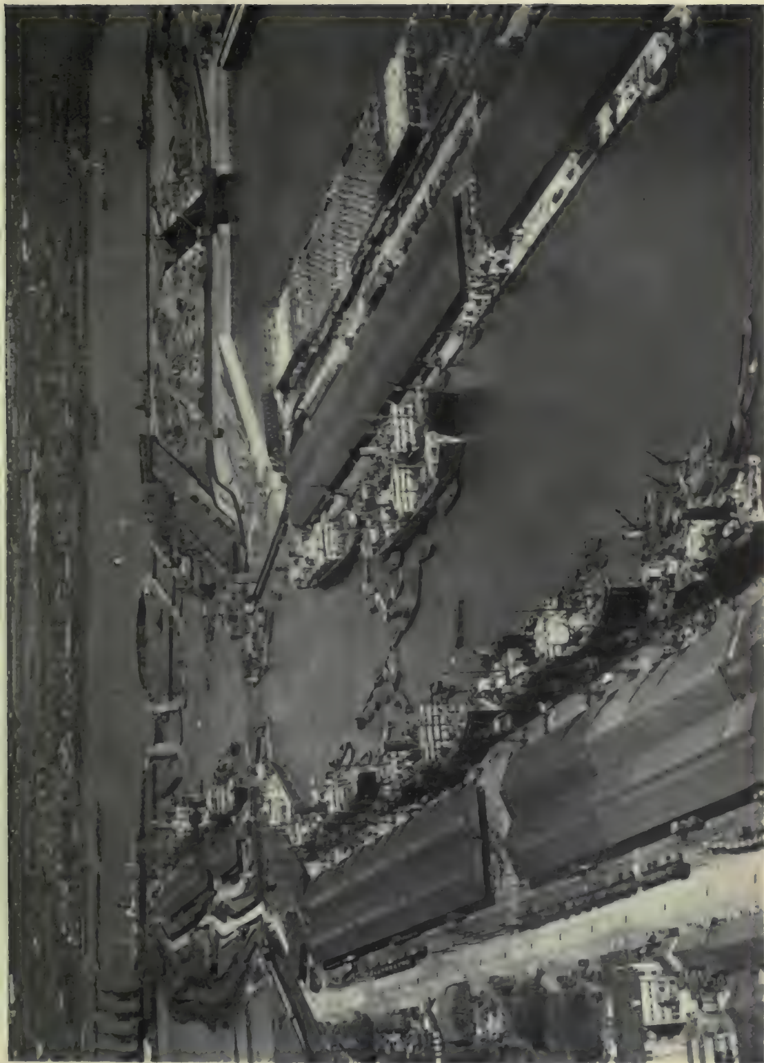
ROYAL ALBERT DOCK From a photograph by the Aircraft Manufacturing Co., Ltd.
