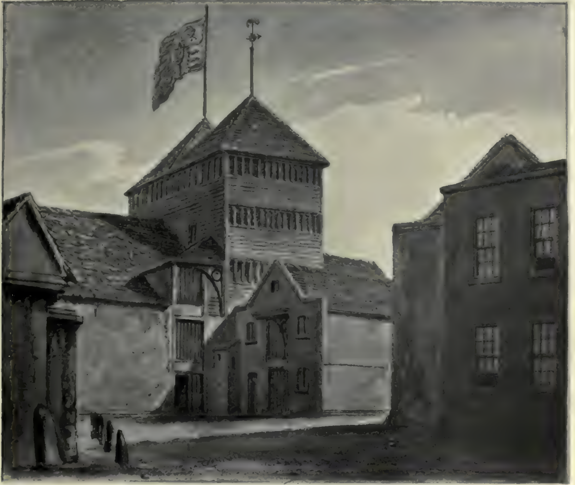
OLD WOOL WAREHOUSE AT BERMONDSEY
